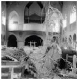
Figure 8: The 1946 earthquake of Siere: Photographs of the collapsed ceiling in the church of Chippis and of the landslide off the Rawylhorn, triggered by an aftershock of the earthquake, as well as a map of the inferred macroseismic intensities.
